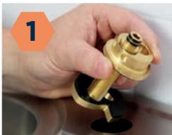
1 Slot the Easyfit base into the sink, insert the hot inlet connector and fix to the sink.
