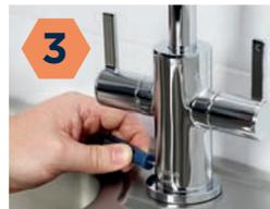
3 Push the tap body on and tighten both grub screws to finish.
